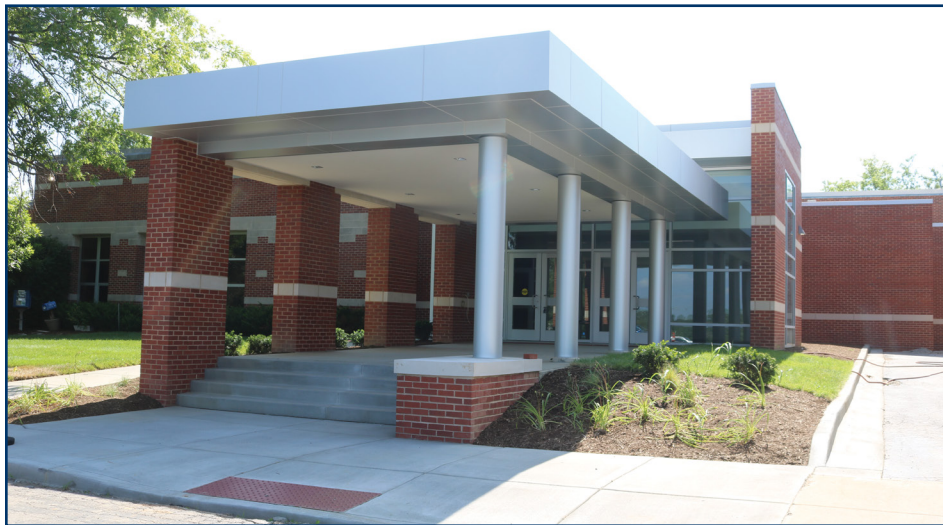
Students will return to Blades Elementary School in August to find a new security entrance and reconfigured front office space.
