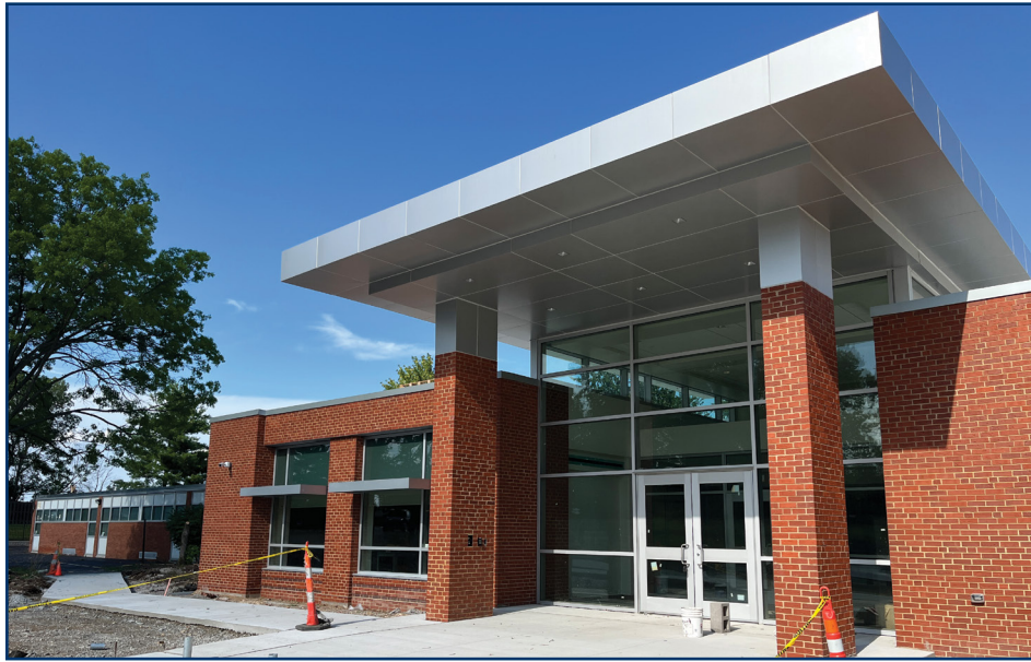
Bierbaum Elementary School has a new secure entrance, reconfigured office space, accessible classrooms and a safer front parking lot configuration. Crews have started work on more classrooms, an expanded library and storm shelter.
