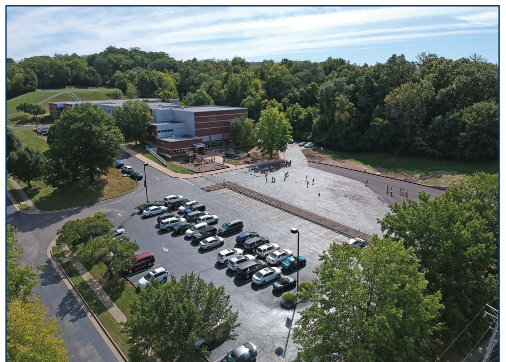
A concrete barrier now separates the Rogers Elementary School parking lot and playground.
