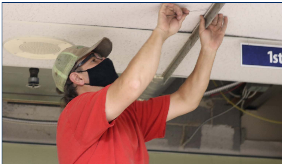
Forder Elementary underwent a complete HVAC renovation this summer.
