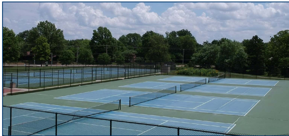
Crews repaired cracks in the tennis courts at Bernard Middle School this summer. The courts were also repainted and new nets were added.
